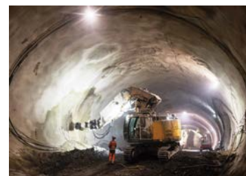
Tunnel construction (concrete spraying)
